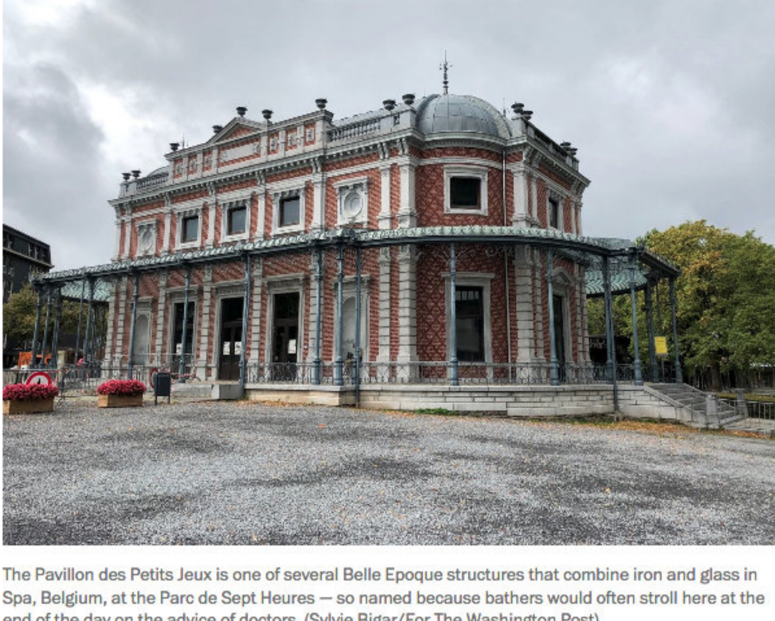
The Pavillon des Petits Jeux is one of several Belle Époque structures that combine iron and glass in Spa, Belgium, at the Parc de Sept Heures — so named because bathers would often stroll here at the end of the day on the advice of doctors. (Sylvie Bigar/For The Washington Post)
